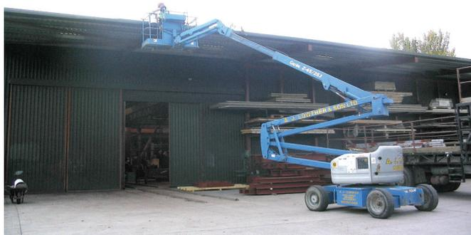
**Figure 4 Using a MEWP to clean the gutter**
