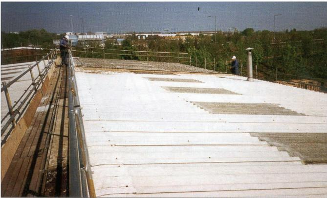
**Figure 1 Complete overlidding of an AC roof**
