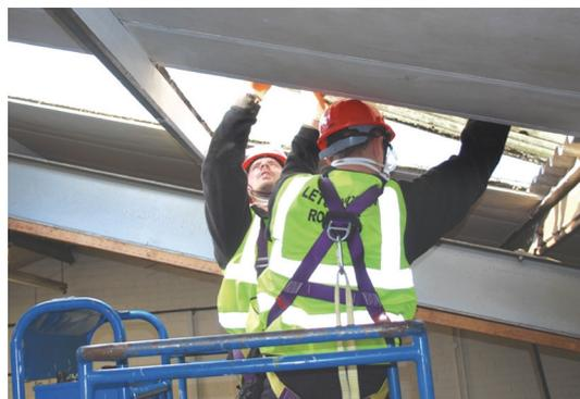
**Figure 6 Replacing a roof light from a MEWP from inside the building using proprietary under roof sheet replacement system.**
