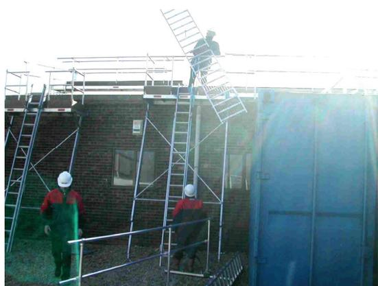
**Figure 3 Installing a proprietary edge protection system**
