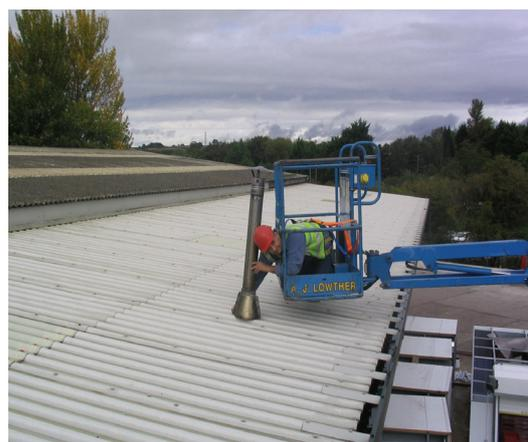
**Figure 2 Using a MEWP to inspect a vent**
